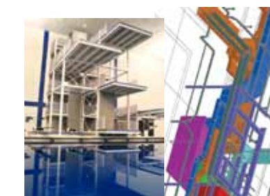
Building Information Modeling was used for shoring of the concrete decks for the dive tower platforms and to provide a layout for support beams. The shoring was built to support the concrete formwork for the platforms.
